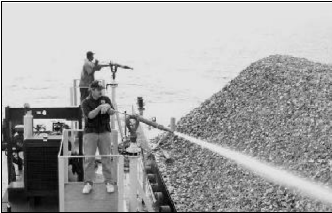
DMR Shellfish Program Coordinator Scott Gordon (front) operates one of the high pressure hoses, used to deploy cultch material on the designated oyster reef site. The DMR distributed nearly 3,950 cubic yards of shell material Sept. 5, about five miles south of Pass Christian.
