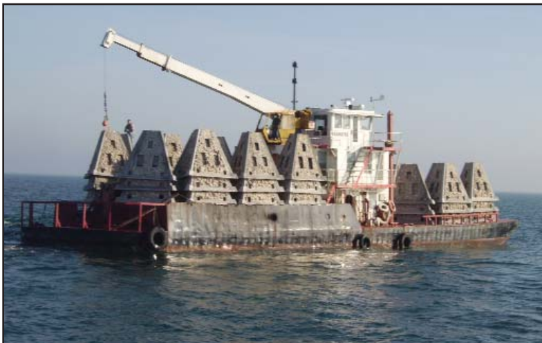
Florida Limestone artificial reefs are transported to Fish Havens 1 and 2, located about 25 miles south of Biloxi.
