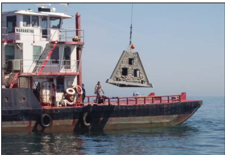
A Florida Limestone reef is hoisted and ready for deployment.
