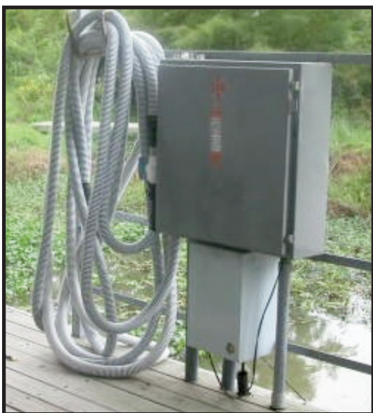
A stand-alone unit is hooked up to the hydrant at a dock using a slip-to-slip pump-out.
