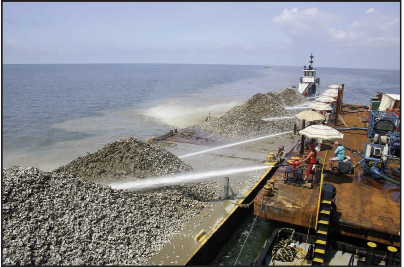
High-pressure hoses are used to spread oyster shells south of Pass Christian in August 2008 as part of the effort to rebuild Mississippi oyster reefs.
