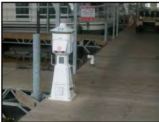
A standalone slip-to-slip pump-out unit provides boaters with a convenient method of pumping out.
