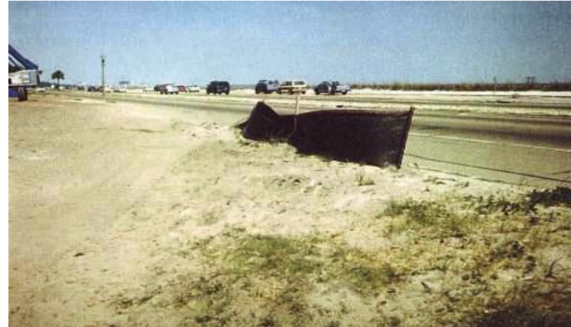
11. A silt fence shown above is a method of trapping fine sediment and sand at a construction site, preventing erosion.
