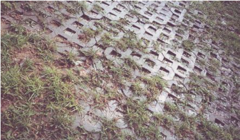
12. This is a grid pavement, a fairly new method of trapping water so that it may filter and percolate through soil, thus some pollutants are absorbed.
