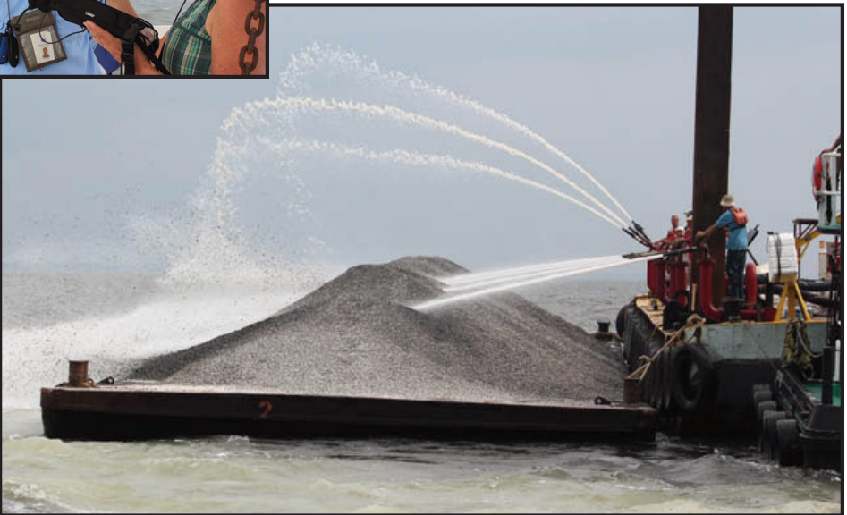
Contractors deploy limestone cultch material to restore oyster reefs in the Mississippi Sound. MDMR's Shellfish Bureau Director Scott Gordon is interviewed by Rhonda Miller with Mississippi Public Broadcasting about the procedure and its importance.
