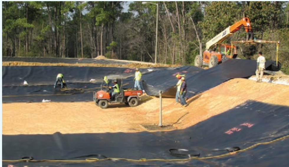
Environmental Specialties International Inc. personnel install new liners at the MDMR Lyman Fish Hatchery.
